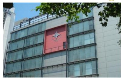
A 9 storied steel framed structure is built on a raft foundation to accommodate offices and a double height studio for MTV channel (Pvt) Ltd. The building is covered with a double skin glass facade.
